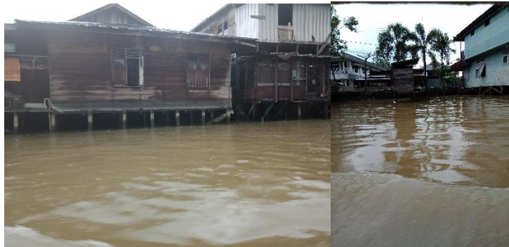
Figure 5. The condition of the houses on the banks of Kuin River (source: Field Documentation, 2019)
