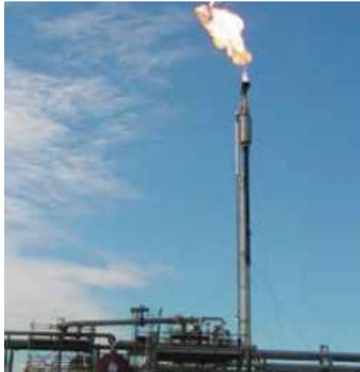
Gambar 1. Instalasi flare stake kilang PT. Pertamina RU V
