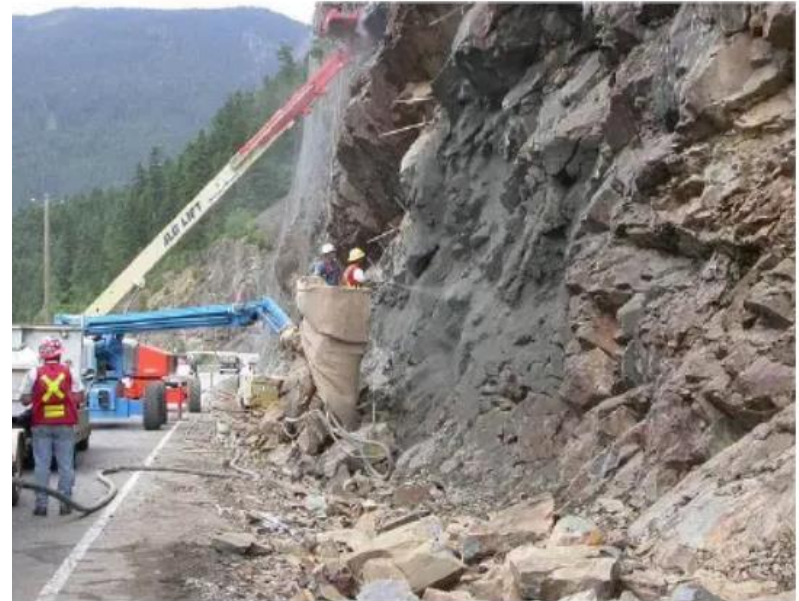
Gambar 2. Pelaksanaan penyemprotan beton shotcrete (sumber : http://www.flickr.com/photos/tranbc/6386097393/ )
