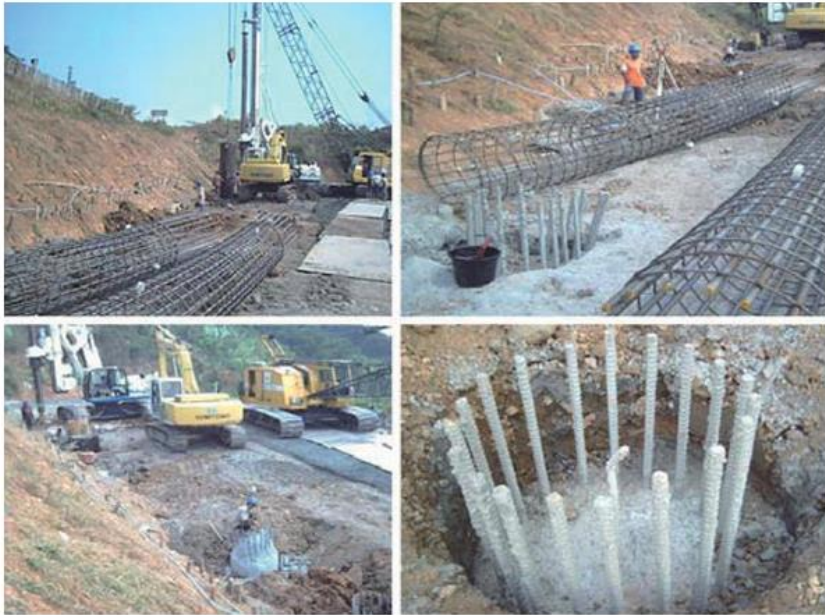
Figure 10 Slope conditions: (a) during construction of bored piles and (b) after construction completion of soldier-bored piles
