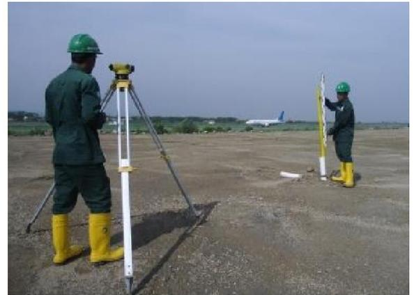
**Gambar 42.** Monitoring *settlement plate*
