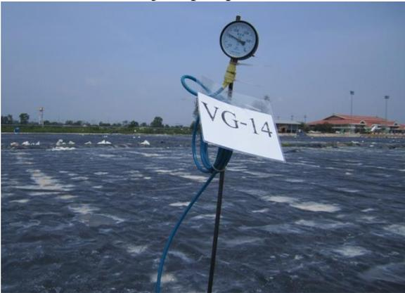
**Gambar 69.** Pekerjaan monitoring *vacuum*
