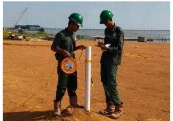
Gambar 67. Monitoring open standpipe pm .
