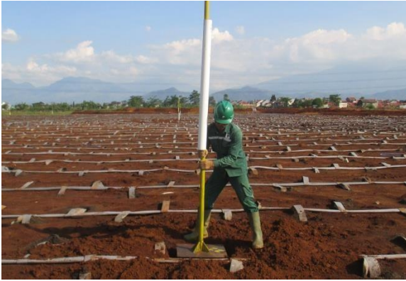
Gambar 50. Pemasangan settlement plate
