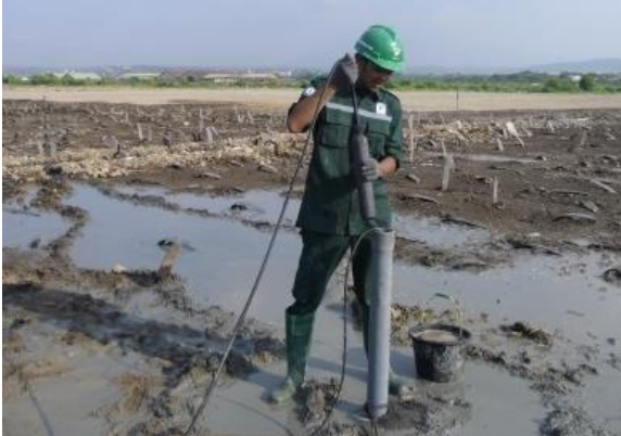
Gambar 52. Pemasangan open standpipe pm.
