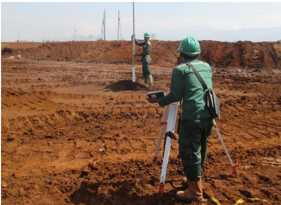
Gambar 58. Monitoring settlement plate
