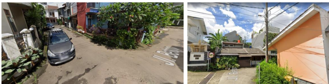
Figure 1. Condition of Intersections and Electrical Cables in Pondok Karya Village
