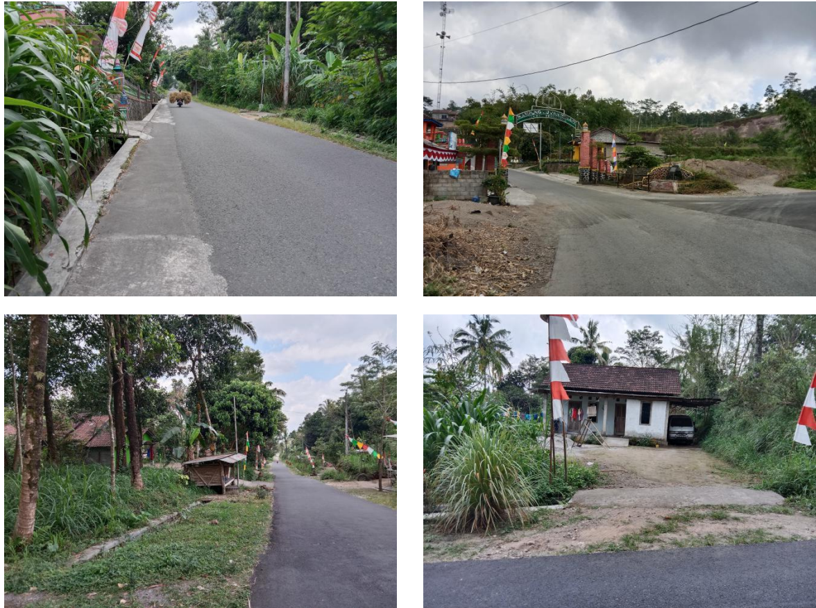
Figure 5. The settlements condition, Source: Field documentation, 2021
