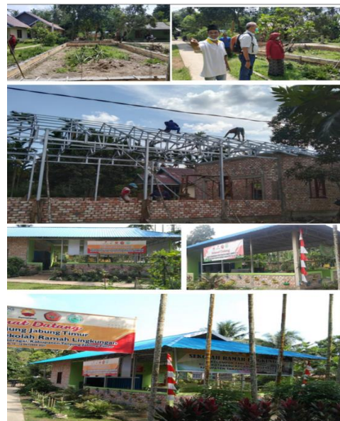
Figure 2 Environmentally friendly school construction
