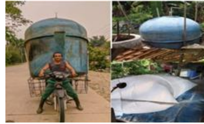
Figure 7 Biogas installation repair
