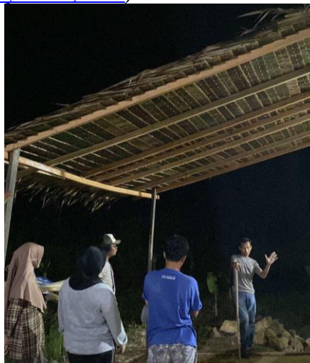
Figure 3 Mushroom house building process
