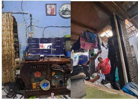
Figure 9 Configuration on the monitor screen and CCTV cable extension
