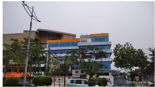
Figure 5 The current Customs Building
