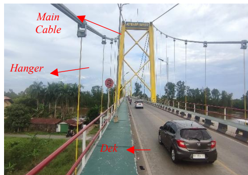
Figure 2. Barito Bridge Structure components
