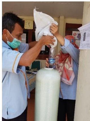
Gambar 5. Persiapan instalasi filter air
