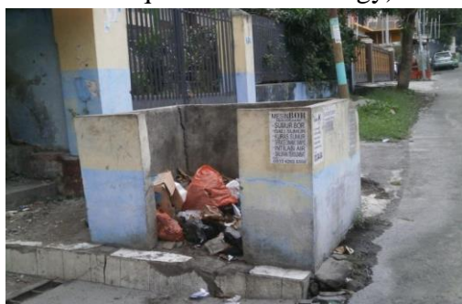
Figure 2. Concrete trash can
