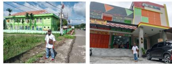
Figure 5. Existing Condition of Building Height
