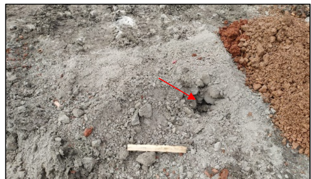
Gambar-3. Lubang ledak tertimbun material
