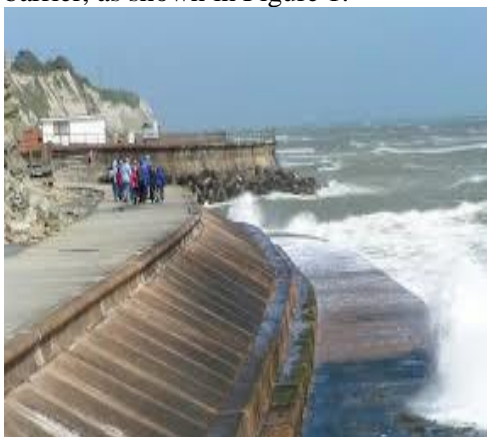
Figure 1 Breakwater on the beach
