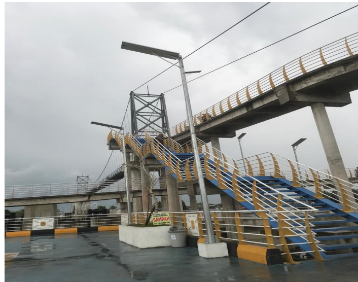
Figure 4. Stairs for Pedestrian Access
