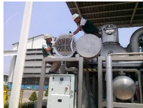
Gambar 10. Perawatan heat exchanger air limbah
